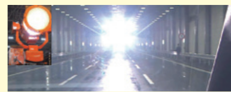
日照設備での点灯状況 Operational situation of sunlight device
